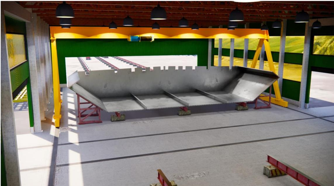
5. Install the top deck (two pieces, temporary structures at beam ends not shown)
